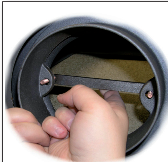
Fig. 7 Affix the flue outlet to the back of the stove using the bolts from the top.
