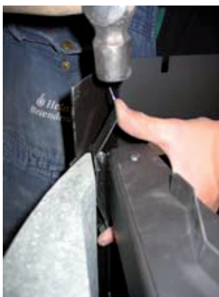
13. Install the spring for the top stone.
