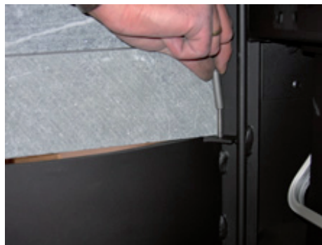
38. Once the stone is in place, carefully re-tighten the screws so that the stone cannot move.
