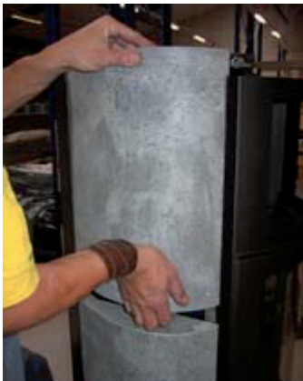
12. Install the top stone.
