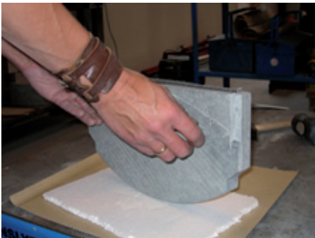
21. Protect the stones during installation.
