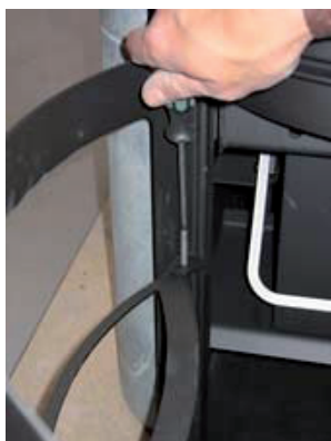
36. Loosen the screw before installing the vertical stone in the ash door.
