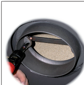
Fig. 8 Make sure that the flue outlet is centred and then tighten the bolts.
